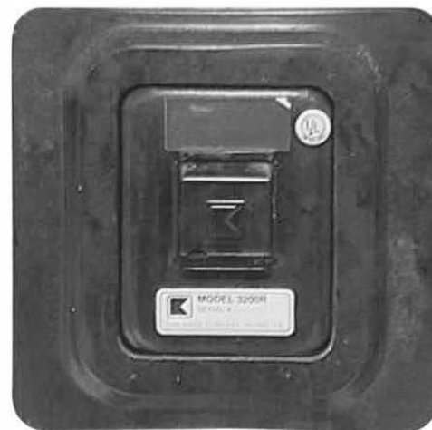
FIGURE 6.5.8.1 Typical Access Box.
